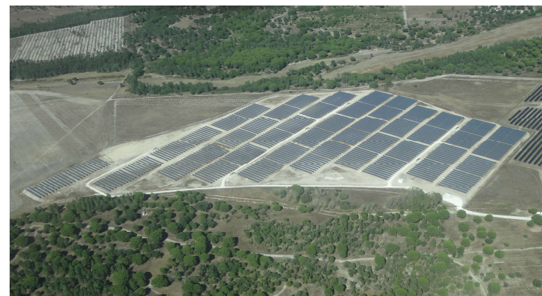
Coruche PV power plant
